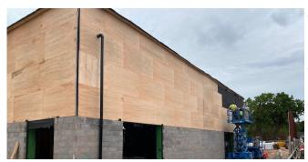
The building is taking shape with most of the triple glazed windows now in place. These take 2 to 3 days to fit for each classroom due to their size and weight! The wooden panels are being fitted to the top half of the building now ready for more insulation next week. This helps to fully insulate the building like a thermos flask for our Passivhaus status. These will then be rendered.
