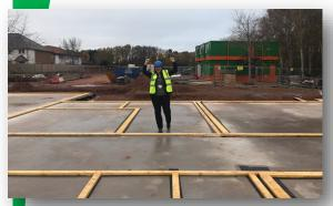
**New Build** I was very excited to be invited to the new build site for our future school last week. The ground works are complete with insulation having been installed. The batons for each of the internal walls have been fitted and the timber frame was due to be delivered yesterday. Please also see the article from
